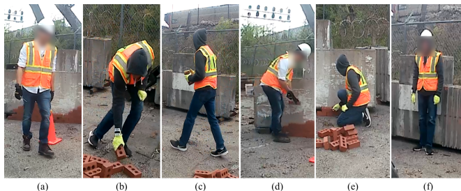
Figure 2. Examples of target activities; (a) walking without a brick, (b) lifting a brick, (c) carrying a brick, (d) placing a brick, (e) tooling, and (f) being idle.
